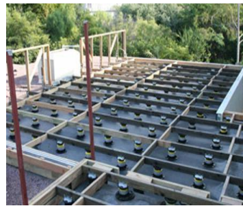
SilcaGrates™ on pedestals with joist adapters and joists. (reduces required number of pedestals.)
