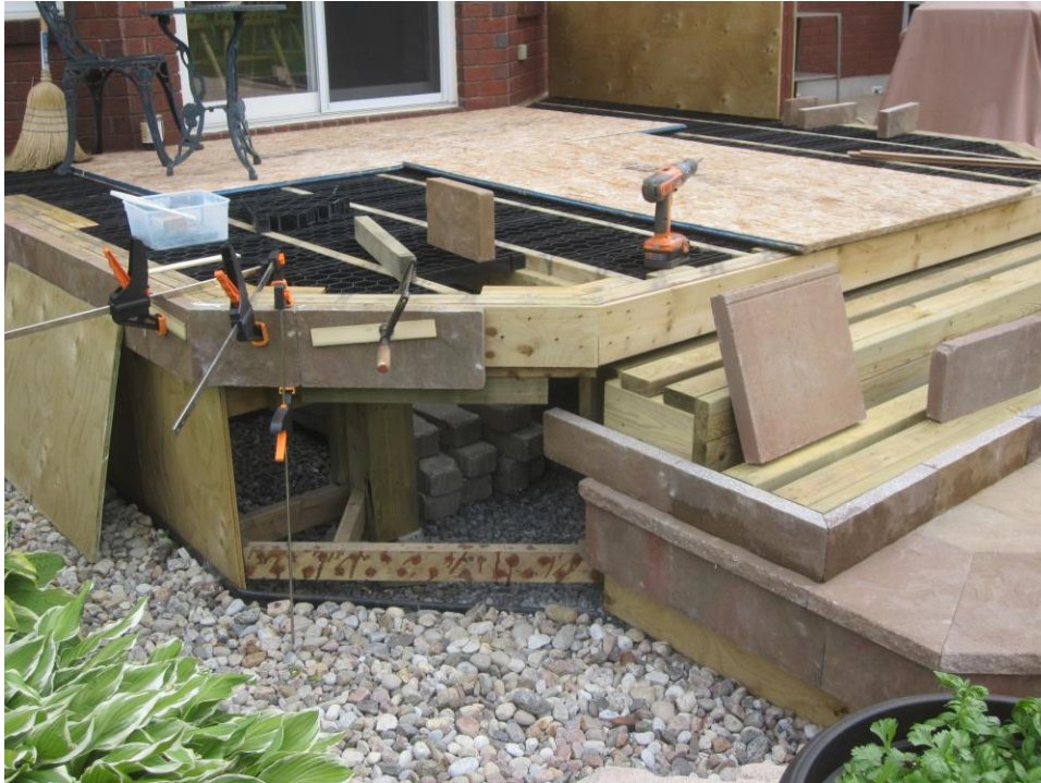
Deck in construction using weatherproof plywood to create a wall for stone veneer.
