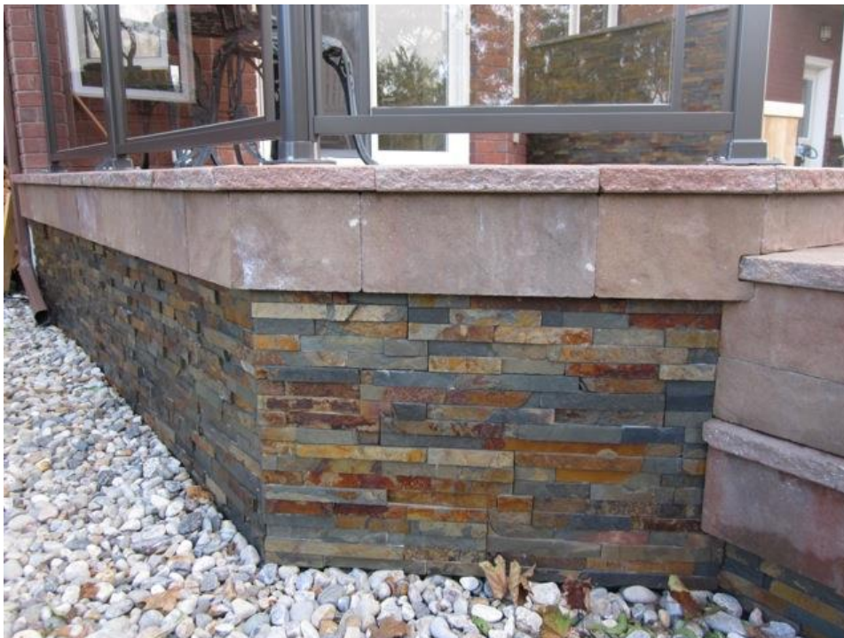
Finished deck and wall. Be sure to allow for ventilation under deck.
