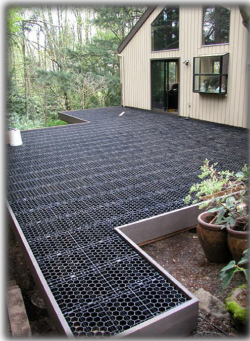
Figure 4 Installed Silca Grates
