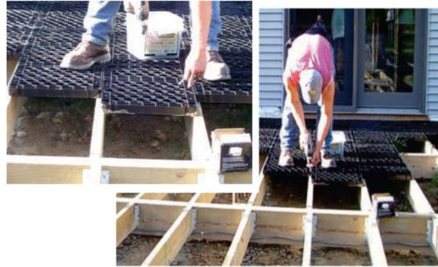
It is recommended that the Silca Grates™ be staggered to achieve maximum strength and stability. To accomplish this start one row of Silca Grates™ with a full grate, and start the next with a half grate.
