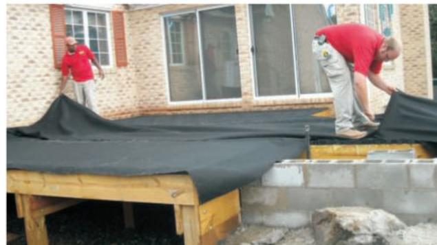
5. Treated Lumber Border – Use a wider dimension lumber for your rim joist (i.e. Use 2x12 for rim joists if your standard joists are 2x8). Generally, you will want the width of the rim joist to be greater than the width of the standard joist by at least the same amount as the combined height of your pavers and Silca Grate™.
